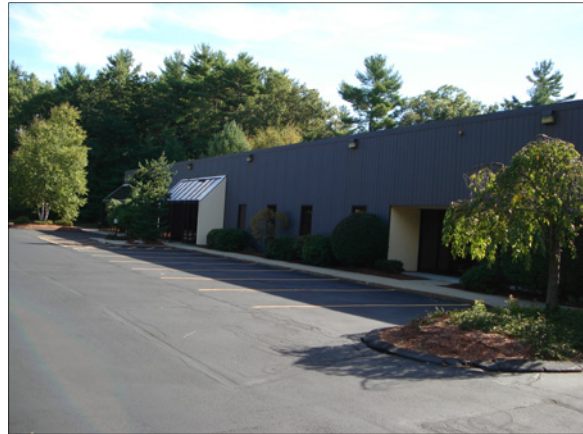
17 Clinton Drive— Front Building View
