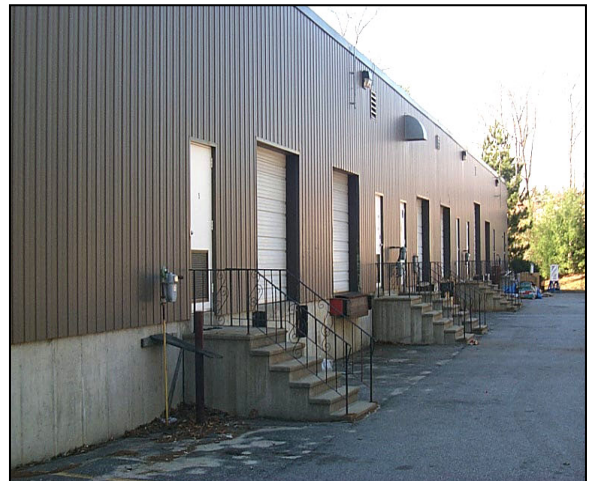
19 Clinton Drive— Loading Docks
