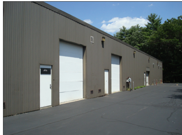
17 Clinton Dr, Unit E drive-in one of two
