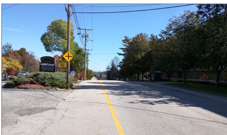
Signage directly on Kinsley Street
